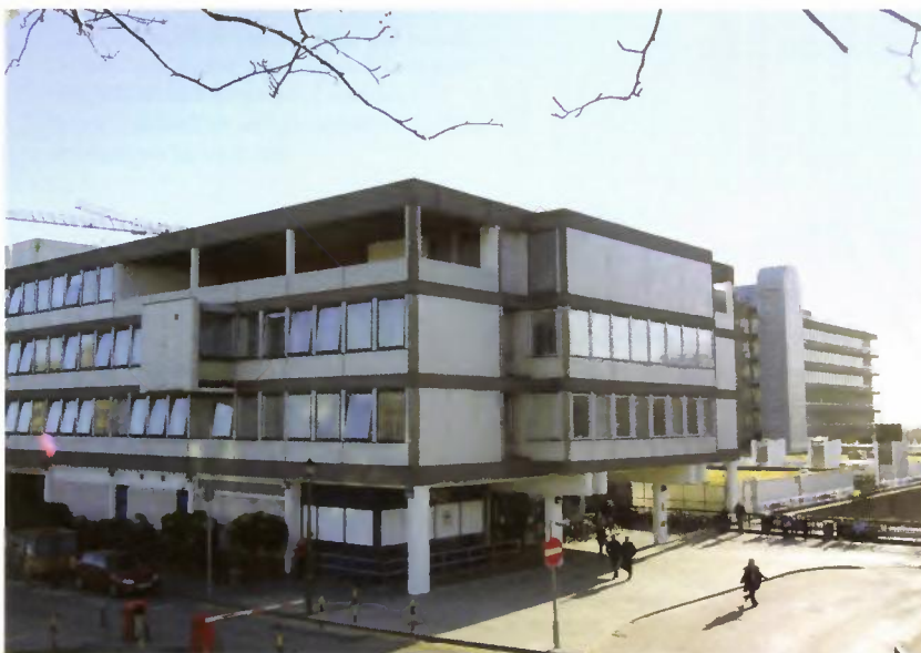
Creating a seamless wireless network in Aberdeen Royal Infirmary meant dealing with a wide variety of building materials, including Cumberland block, sandstone, and even granite
